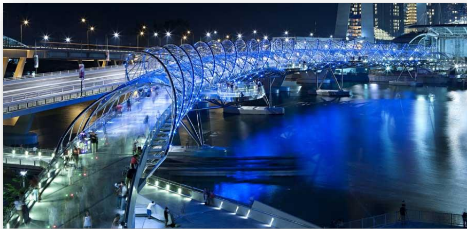
Helix Bridge, Singapore
